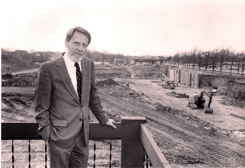
[The big black hole Klaus Schulten observed at the Beckman Institute construction site. Ted Brown, its first director, is in the foreground. Photo courtesy of the Beckman Institute.]
