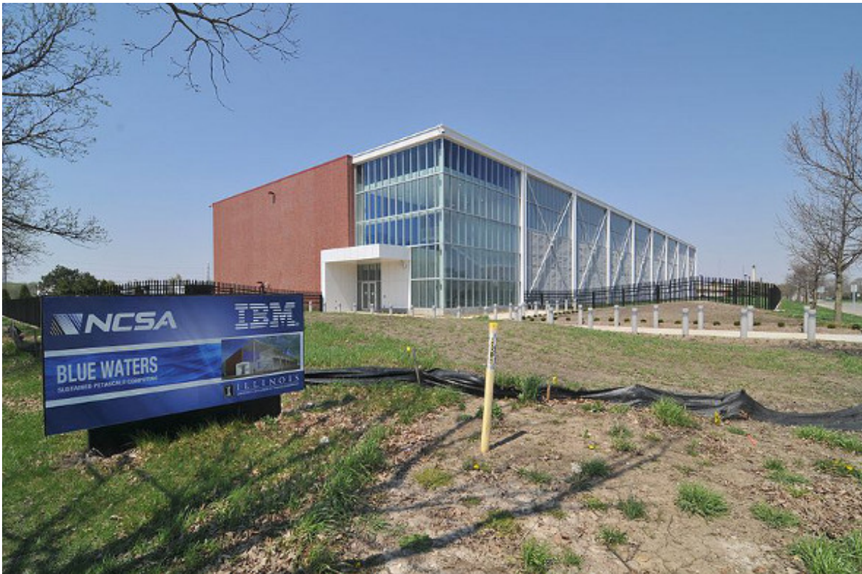
Blue Waters Supercomputing Center at UIUC
